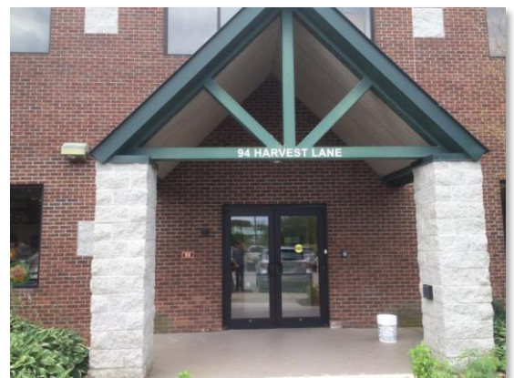
The new office on Harvest Lane in Williston
